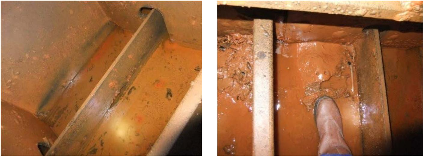
Figure 4 – Drainage arrangements through tank floors (left) and typical sediment build-up reducing the free flow of water between chambers and bays (right)
