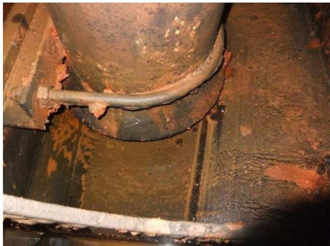
Figure 3 – 'Elephant's foot' forming the pipe opening
