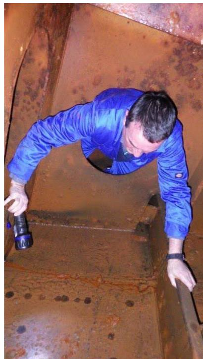
Figure 2 – Tank internal structures create many compartments and chambers linked by openings and drain channels
